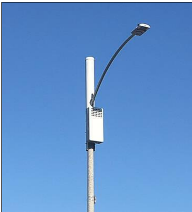
Figure 4: Flush-mounted radio shroud.
